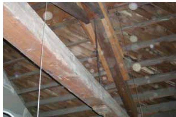
Figure 7 - Repair @ Top Chord
