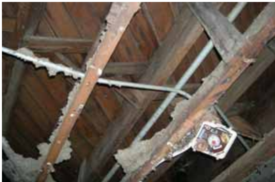
Figure 20 - 2x12 Roof Joists with Suspended 2x's & Remnants of Previous Ceiling
