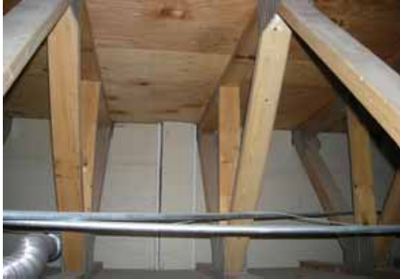
Figure 21 - 2nd Floor Office Gang-Nail Truss Framing
