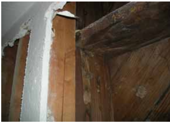
Figure 22 - Interior View of 2x4 Bearing Wall @ Office Truss & Exterior 2x8 Wall
