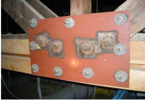
Figure 12 - (n) Steel Plate and Repair @ Bottom Chord
