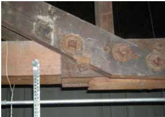
Figure 14 - Bolt not in Diagonal
